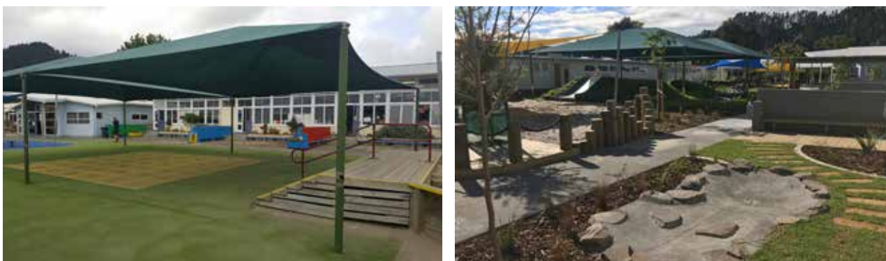
FIGURE 1. STATE SCHOOL 1 BEFORE TRANSFORMATION (L) AND AFTER TRANSFORMATION (R)
